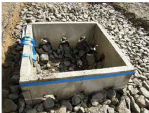
Stones that fall into the foundation openings mean that the foundation is fixed.
