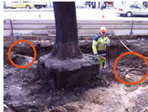
Pipeline roots exposed during excavation.
