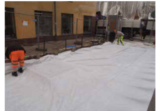
Geotextile extends across the leveling layer and the entire plant bed. It is important that the geotextile folds against tree-pit foundations, wells and edge supports to prevent the pavement bearing layer from being mixed with aerated bearing layer.
