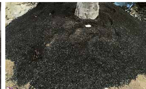
Covering of roots with biochar macadam.
