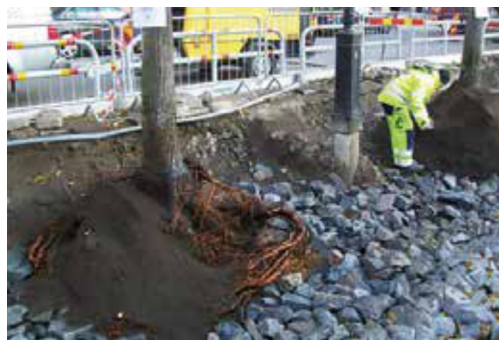
Plant bed renovation on Birger Jarlsgatan.
