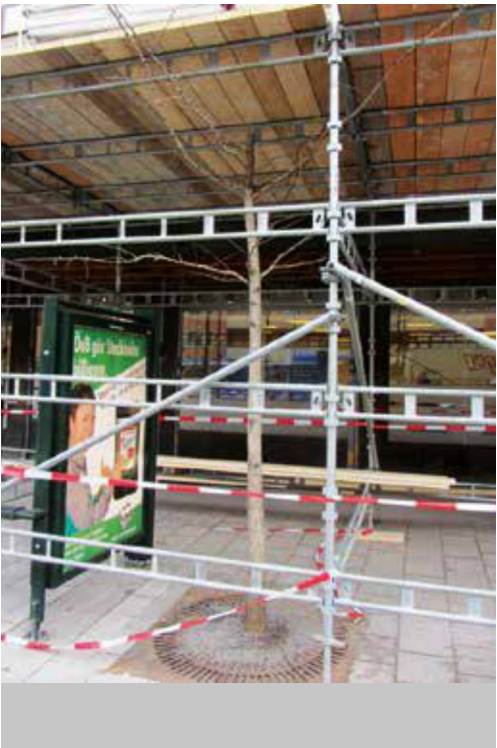
Example of damage: the tree has been sawn when mounting the scaffolding.
