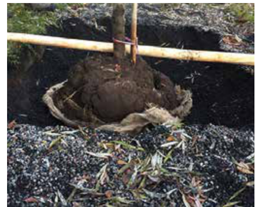
Tree root neck placement at the same level as in the nursery. The height position is adjusted as needed with macadam in the bottom of the tree pit. Photo Lovisa Hell.
