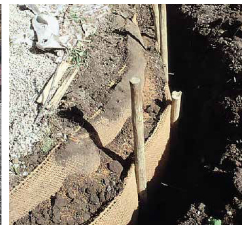
Root drapery of coconut carpet mounted on wooden stakes with moist soil. When backfilling cannot be carried out immediately, the root canopy protects the tree roots from dehydration.
