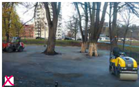
No fencing and no protection against soil compaction
