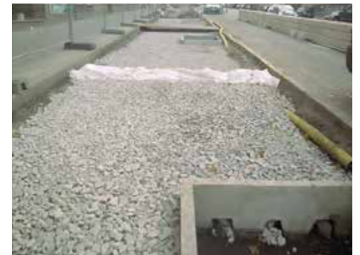
The geotextile dam in aerated bearing layer.
