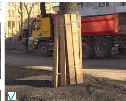
Trees protected with cover and boards for plant bed renovation. Photo Lovisa Hell.
