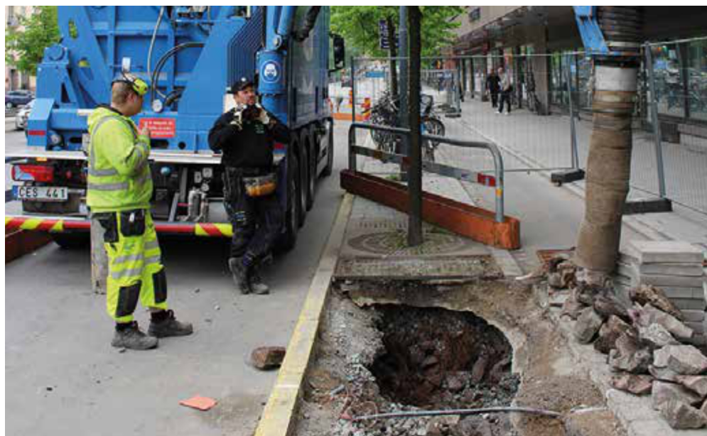
Sample excavation in structural soil for root distribution evaluation.
