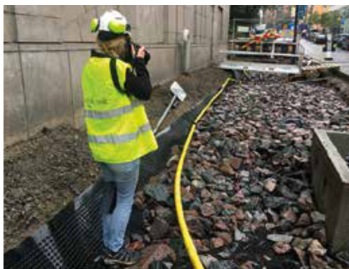
Documentation of watering down of biochar macadam in structural stone layer. Photo Hildegun Varhelyi.
